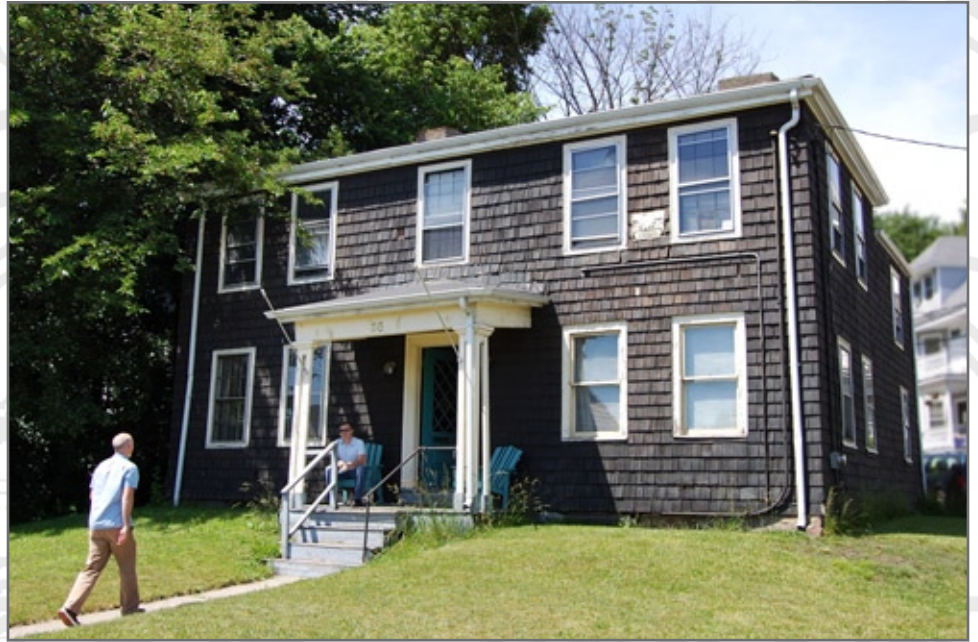
The Anna Clapp Harris Smith House, located at 65 Pleasant Street in Dorchester, was built in 1804 on a foundation that purportedly dates to 1636.
