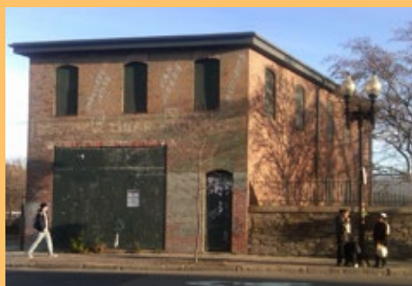
A New Look at Roxbury's Owen Nawn Factory p6
