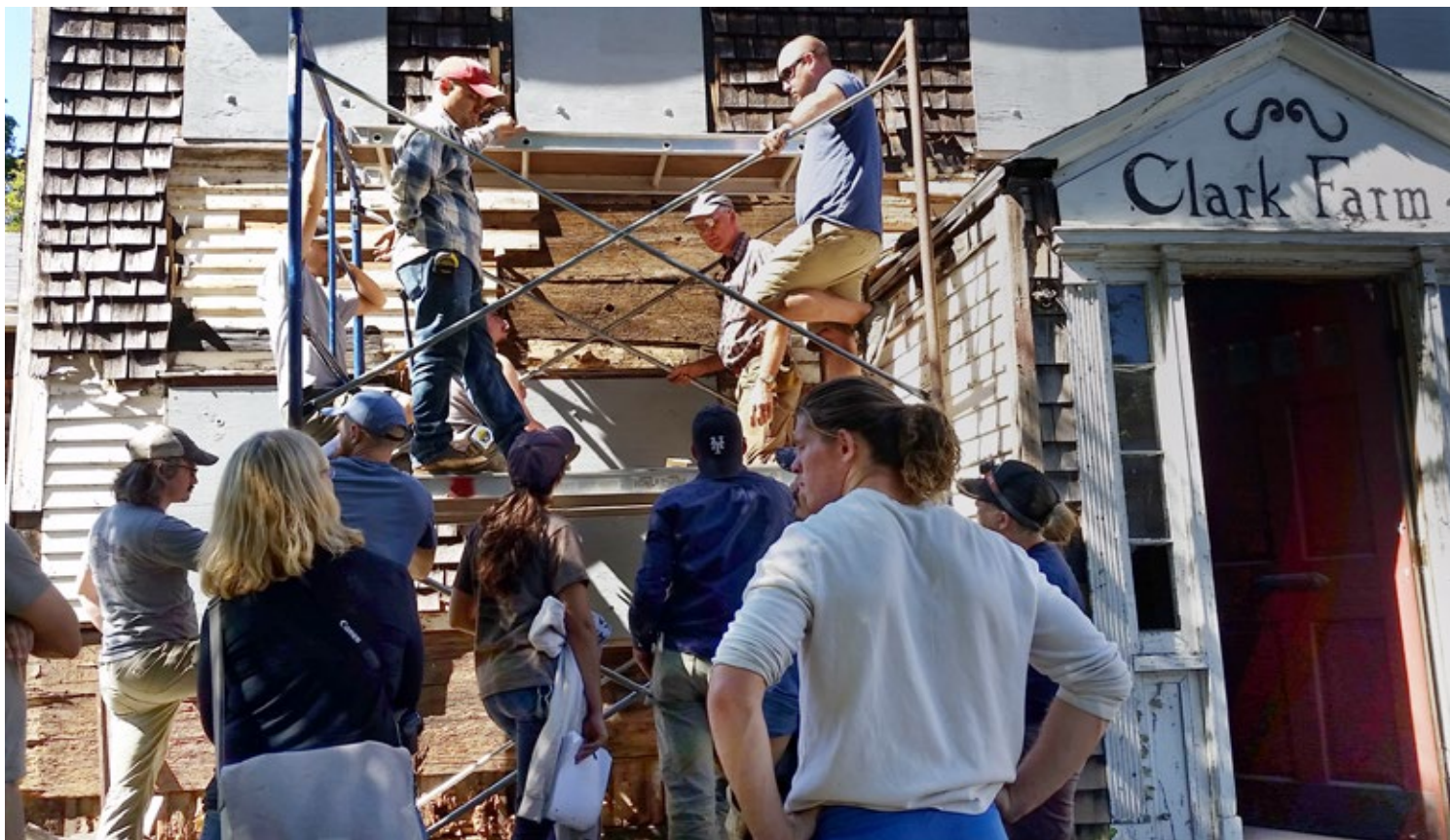
▲ North Bennet Street School's preservation carpentry students conduct exploratory work on the farmhouse.
