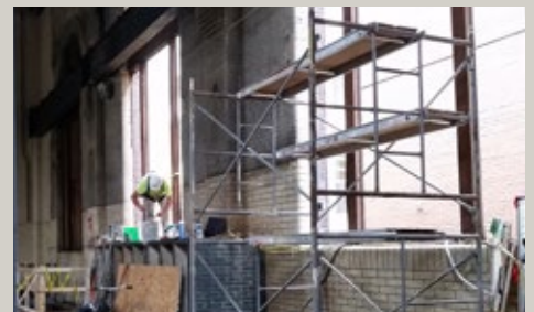
▲ In-fill brick has been removed for window restoration.
