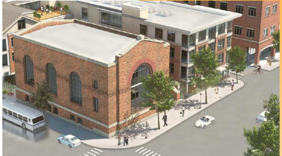
Empty since 1970, the Roslindale Substation is proposed for re-use as a destination restaurant and craft beer retailer.
