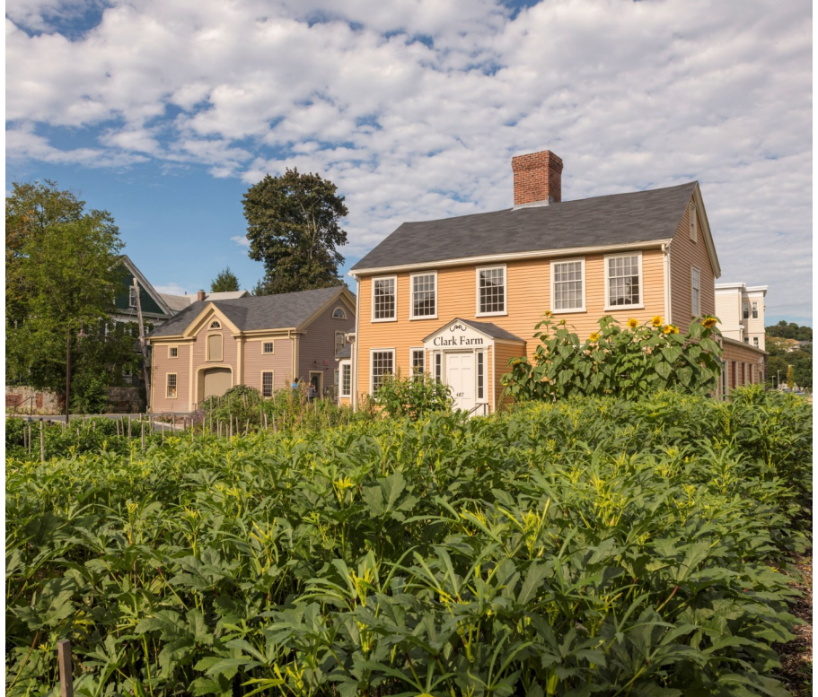
View of rehabilitated Fowler Clark Epstein Farm.
