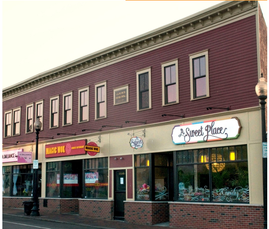
Restored exterior of Roslindale Substation.
