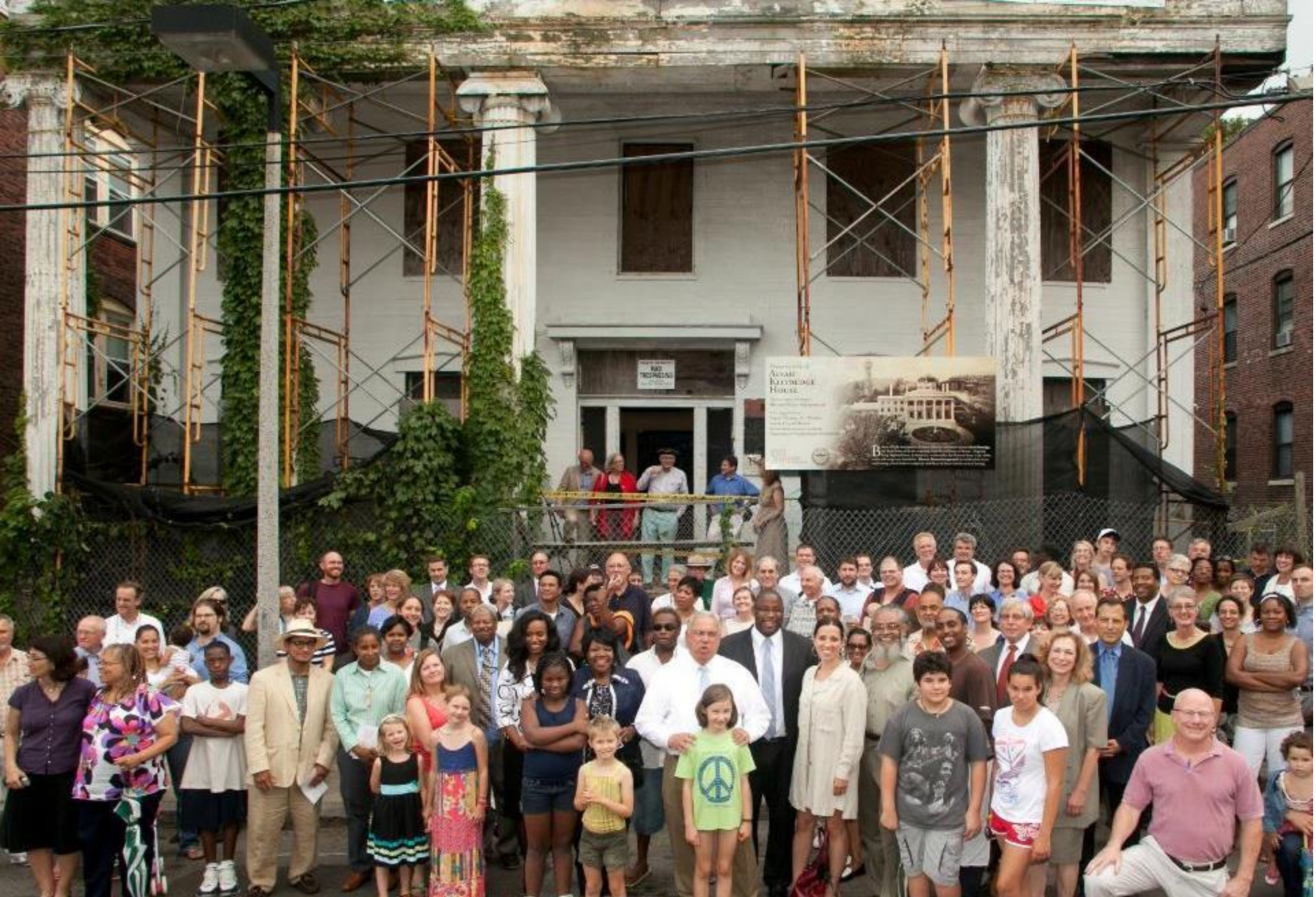
ALVAH KITTREDGE HOUSE (1834) Rehabilitation for Mixed Income Apartments in 2014
