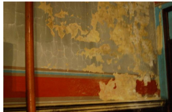
Figure 6 deteriorating historic materials, and example of original paint colors
