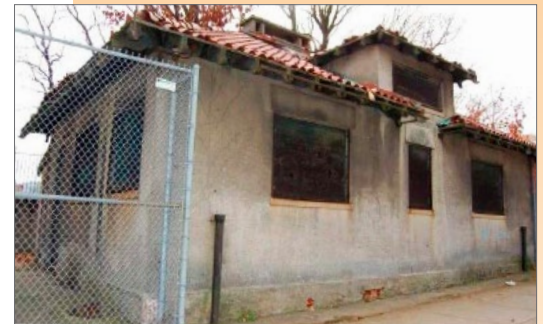
Vacant since 1977, the Upham's Corner Comfort Station is shown before restoration.
