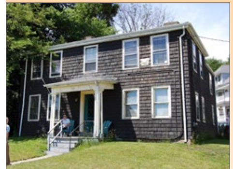
The Anna Clapp Harris Smith house before restoration.
