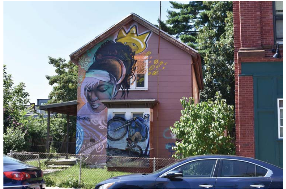
2. 197 Green Street, view southwest.
