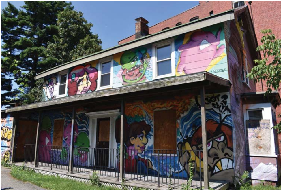
1. 197 Green Street, view southwest.
