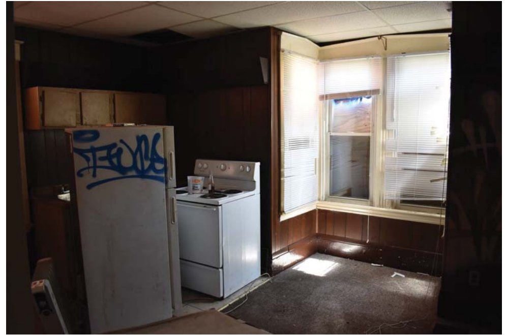
18. Front room on first floor.
