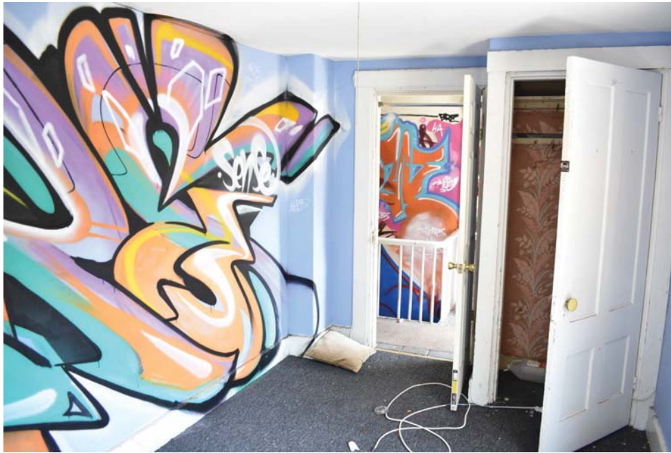
21. Southwest bedroom on second floor.
