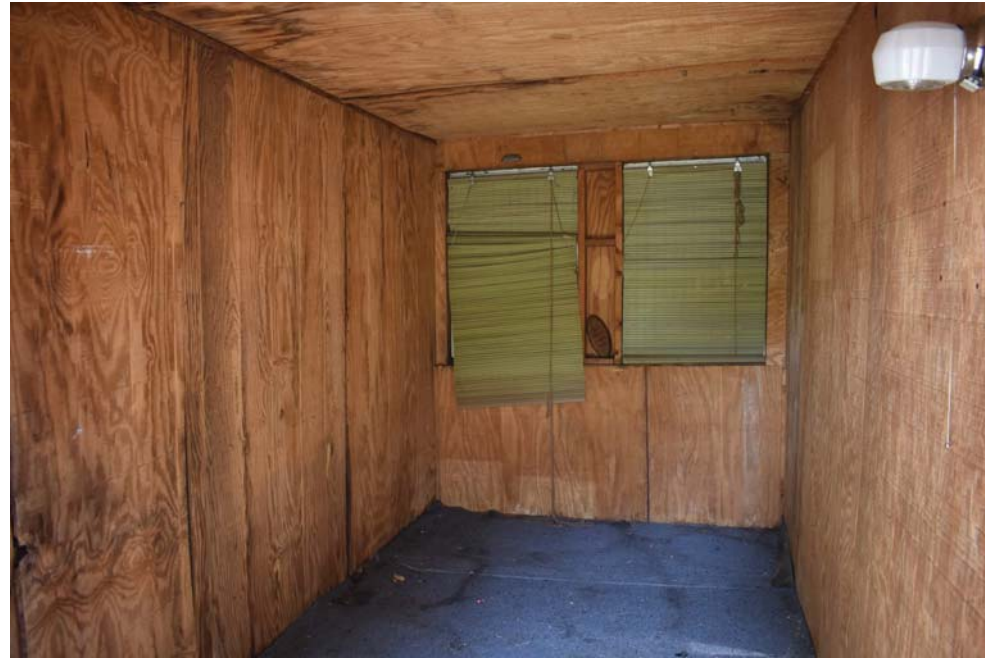
10. Enclosed porch on rear of building.
