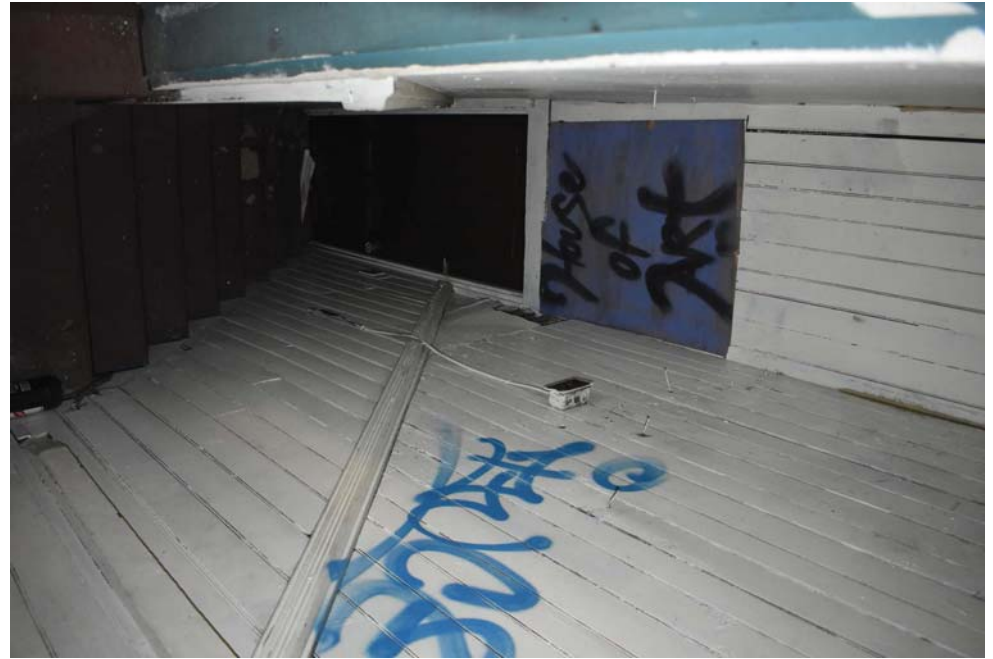
26. Rear staircase from second floor.
