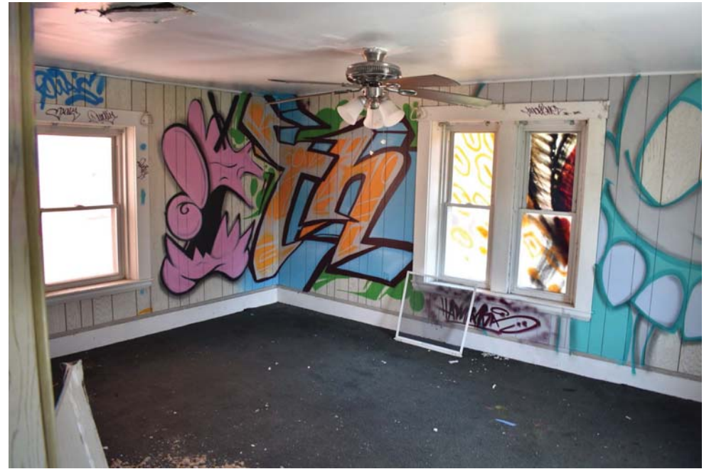
22. Front bedroom on second floor.
