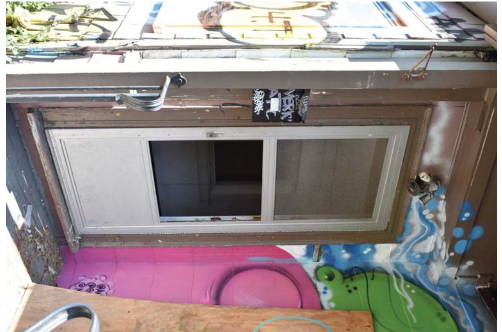
8. Secondary entrance on southeast elevation.
