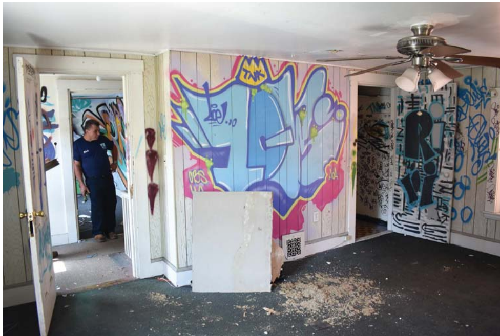
23. Front bedroom on second floor.
