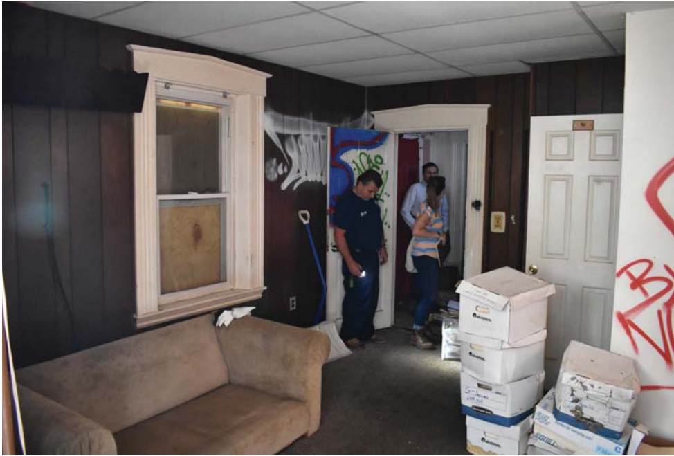
17. Front room and vestibule on first floor.
