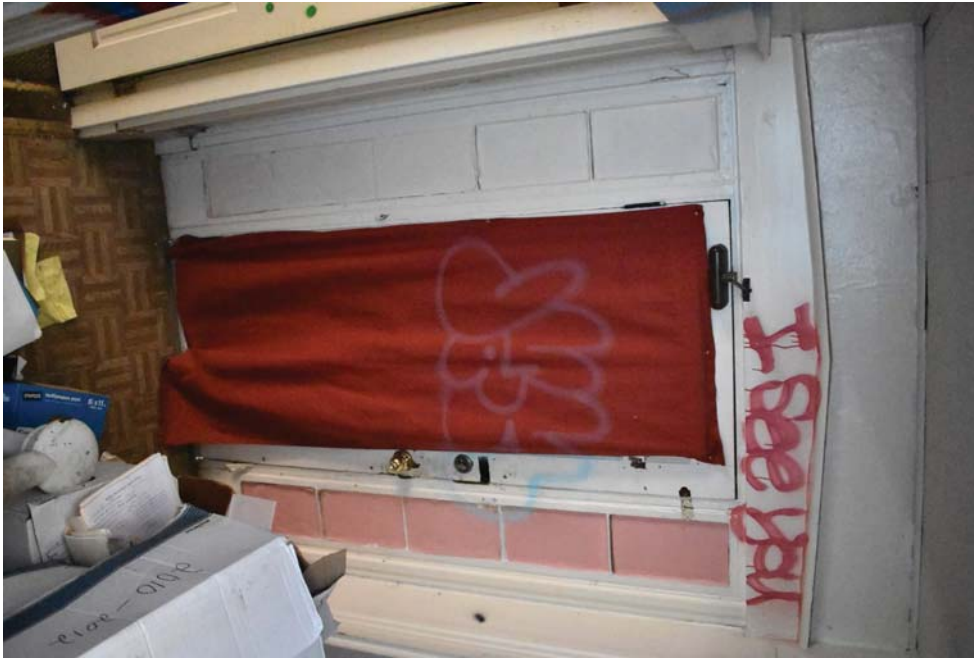
13. Main entrance and vestibule.
