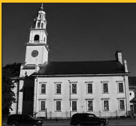
First Parish Church, Dorchester received a grant to repair its badly leaning steeple.
