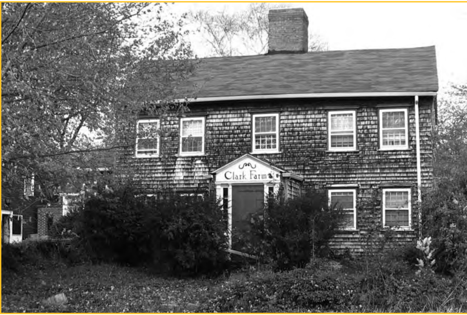
The front façade of the endangered Fowler-Clark Farmhouse.
