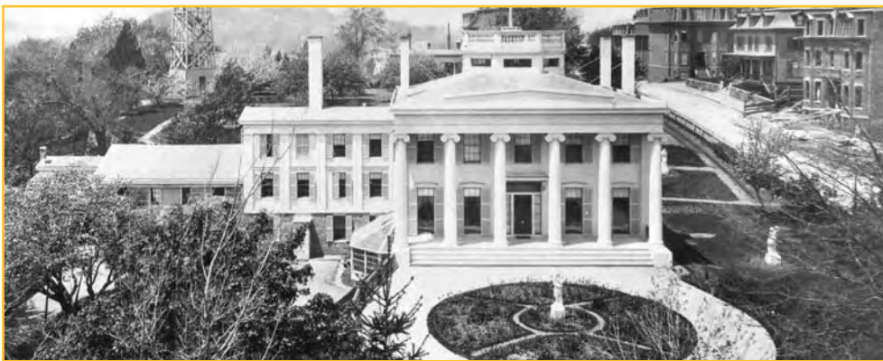
The 1836 Alvah Kittredge House and grounds as it appeared in the 1880s. & ALVAH KITTREDGE HOUSE CURRENT PHOTO - CAPTION: A current photo of the dilapidated Alvah Kittredge House showing the two columns missing from its portico.
