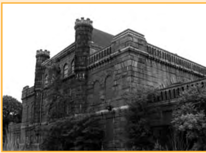
Calf Pasture Pumping Station, Dorchester
