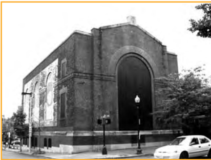
Rosindale MBTA Substation
