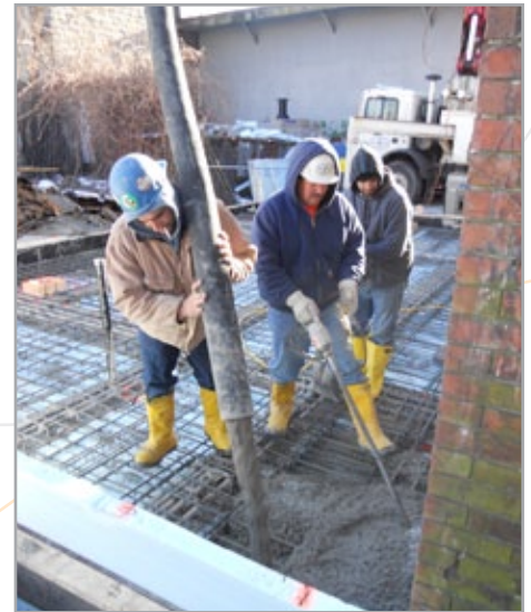
Workers from Lee Kennedy Co. prepare the foundation of an addition at the rear of the firehouse.
